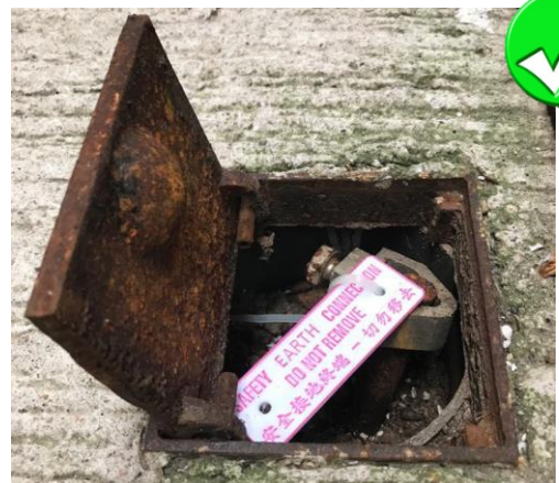
Earth electrode with inspection pit shall be provided.
