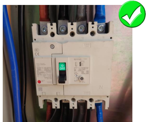
Residual current device shall be provided at customer's LV main switch.
