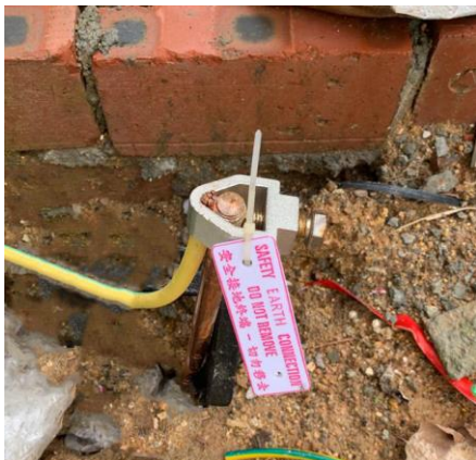
Earth electrode without inspection pit.
