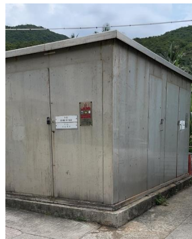
Pre-fabricated modular transformer pillar provided by HK Electric
